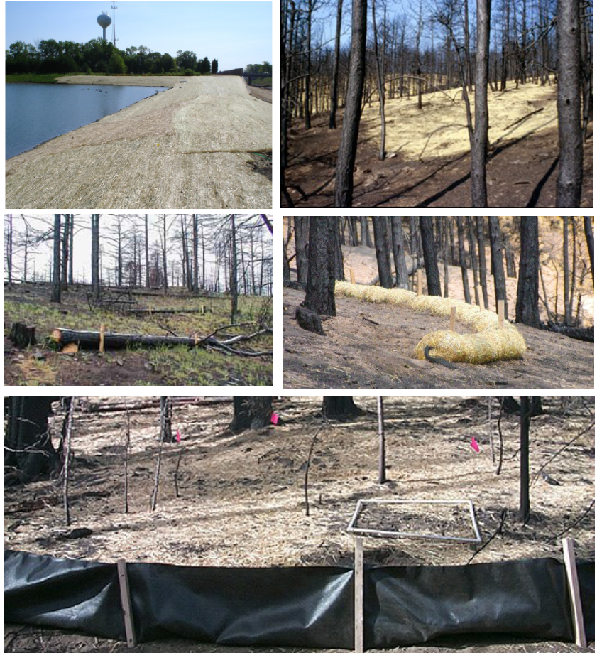
Figure 7. Post-wildfire erosion control methods include mulching, erosion control mats, log terraces, fiber rolls, and silt fences. (Sources: Minnesota Pollution Control Agency, Afterwildfirenm.org, Colorado State Extension, and Moscow Forestry Science Laboratory of Washington State University)
